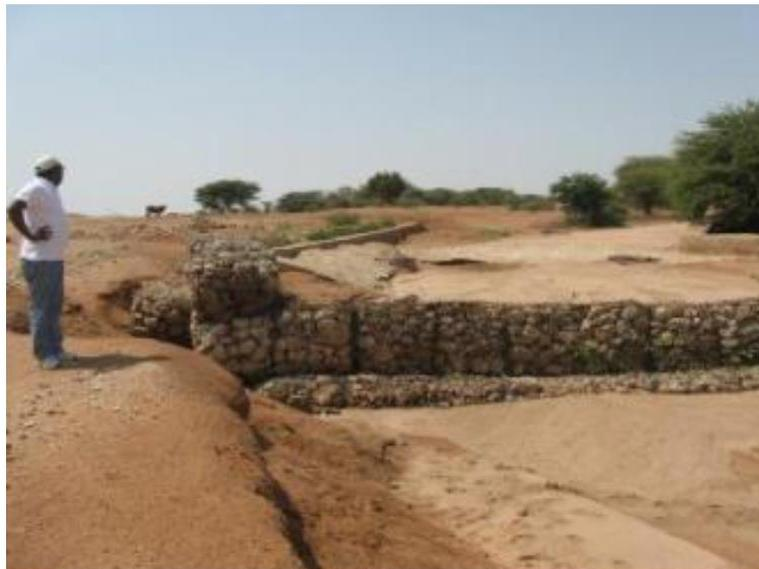
**Figure 11: Subsurface (sand) dams near Hargeysa (photo Z.Stevanovic) (FAO SWALIM)**
